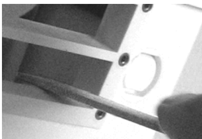
Figure 30: Filing Rough Edges
